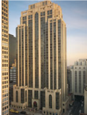
Helmsley Medical Tower - 1320 York Ave.
